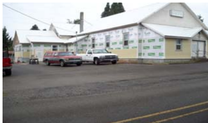
Building wrapped & new siding begun
